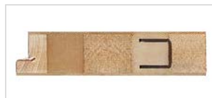
door leaf 46 mm enforcement with massive iron profile
